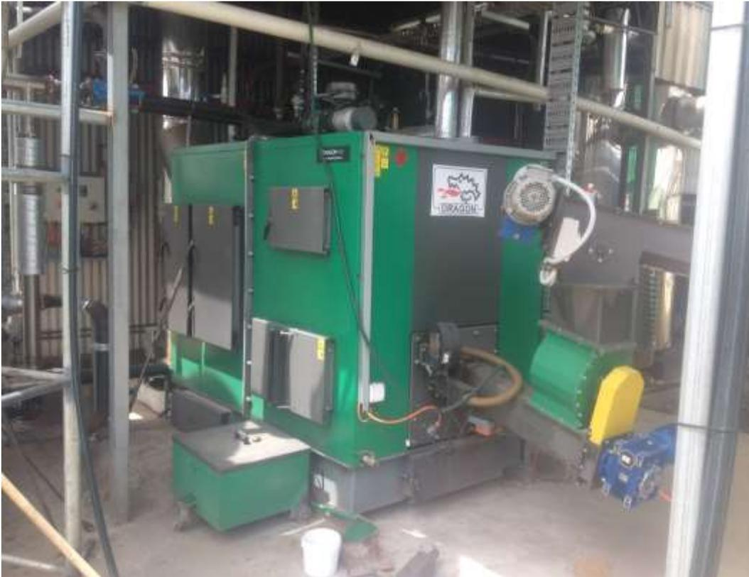
*240 kW biomass boiler at Meredith Dairy provides 85° hot water for food processing. The woodchip fuelled boiler is manufactured by Moderator in Poland.*
